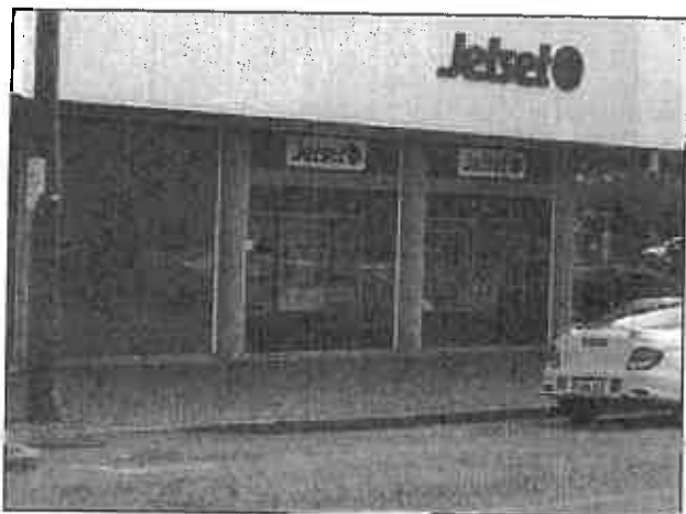
Figure 6 - Example of building facade style that is not acceptable.
